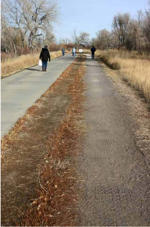
Slight separation between the adjoining treads, one concrete and the other natural surface often used by equestrians; Crown Hill Park trails in Wheat Ridge, CO; photo by Stuart Macdonald, 20 Dec 2010.
