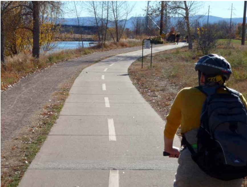
Crusher fines trail marked for pedestrians along Mary Carter Greenway by the Platte River, South Suburban Park District, Colorado; photo by Stuart Macdonald, 7 Nov 2010.
