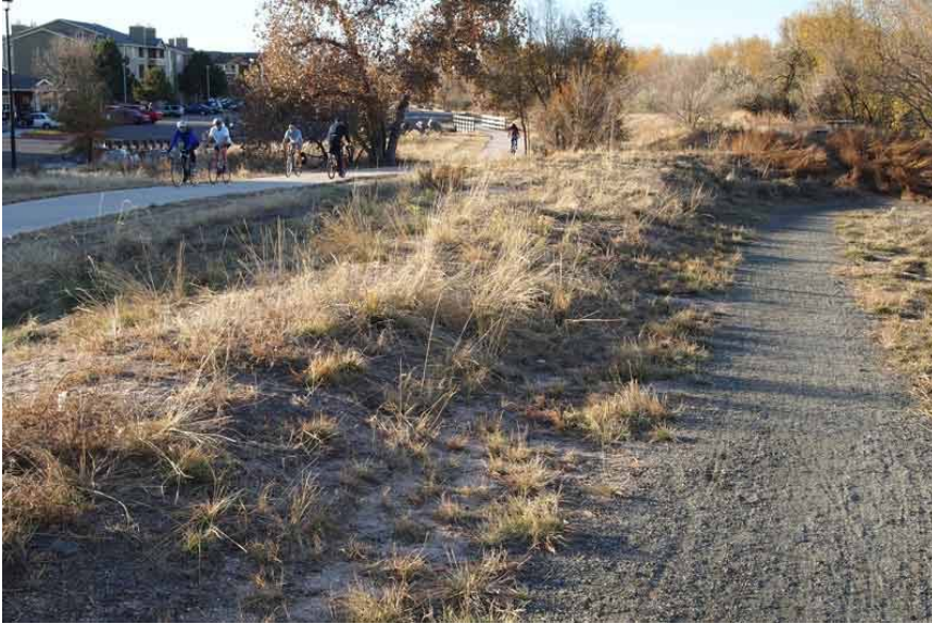
Crusher fines trail is separated from concrete Cherry Creek Trail, Denver, CO; photo by Stuart Macdonald, 6 Nov 2009.
